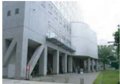
Building of Conference Venue
